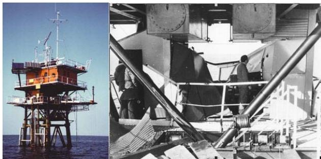
**Fig. 2.** The oceanographic tower of ISMAR in the northern Adriatic Sea, 15 km offshore the Venice coastline. Right panel: the tower (second floor, +7 m a.m.s.l.) after the storm of 22 December 1979. The position of the tower is shown in Fig. 3.
