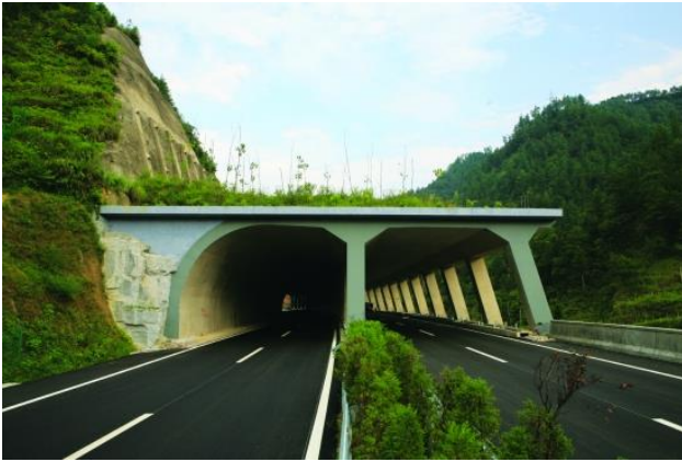
Fig. 1. Rock-shed on the Chongqing to Hunan highway with reinforced concrete columns, foundation and a roof slab; the width of the road for single pass is 8.5 m (Chongqing daily press photos).
